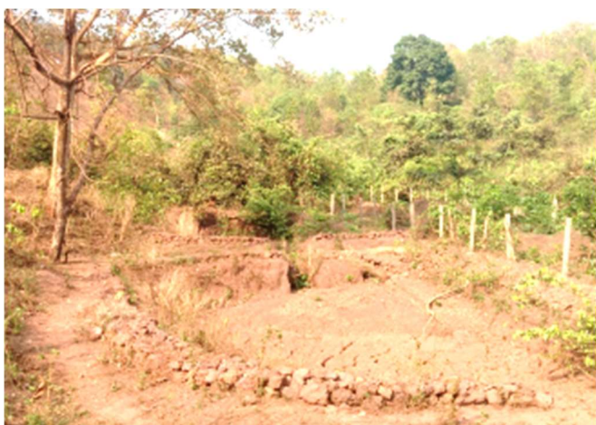
Photo-8& 9: Settling cum water harvesting pit
