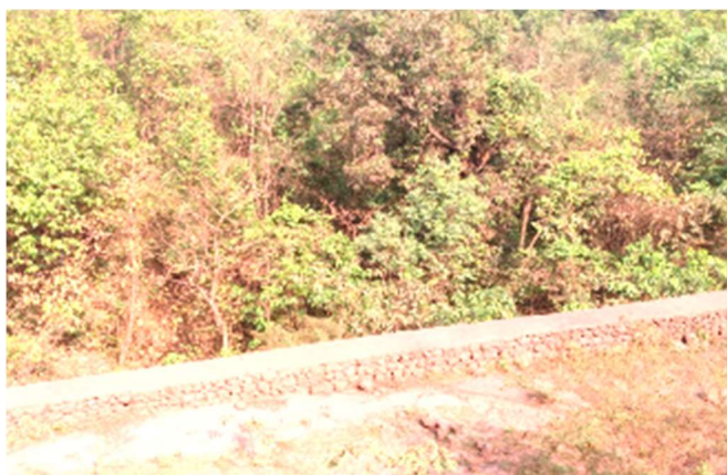
Photo-10: Check Weir
